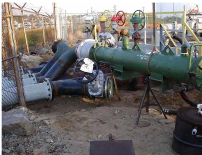
**Figure 1. A single launch and receive location was used with a single temporary barrel. Four lines were cleaned and inspected in less than one week.**
