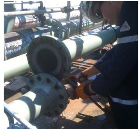
InVista™ being retrieved after flange disassembly. Time to remove InVista from pipe = 15 minutes
