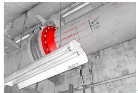
Figure 1. Nozzle and Tie-Point Verification
