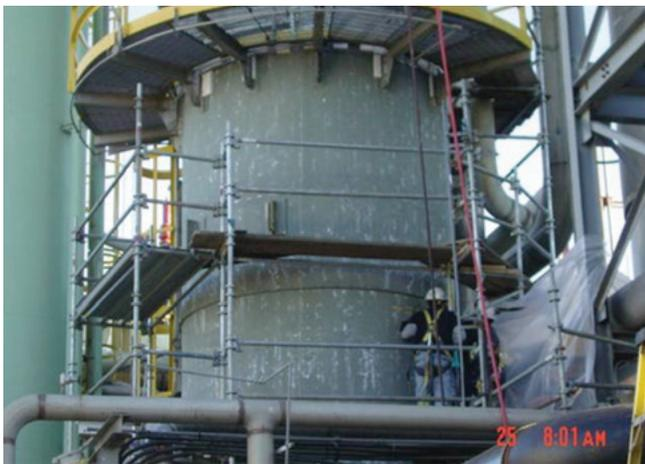
Figure 4 – Monitoring Internal Corrosion Using an External UT Grid
