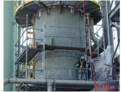
Figure 4. Monitoring internal corrosion using an external UT grid
