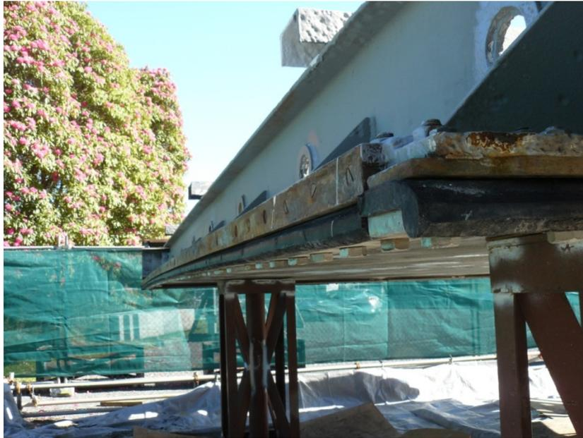
*Figure 1. Deflection at the bottom of spillway gate No. 2*
