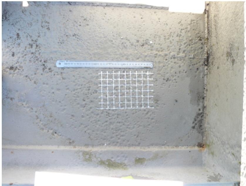
*Figure 2. Surface corrosion in between lower girders A3 and A2*
