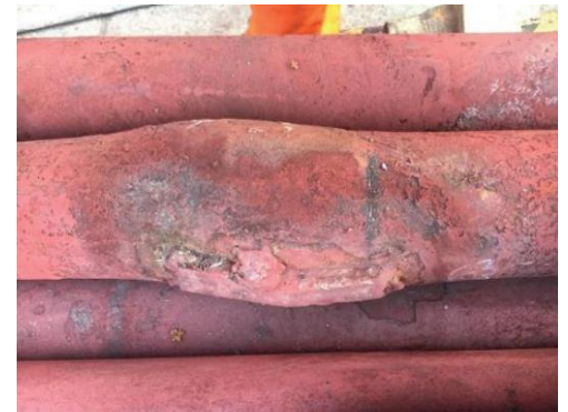
Figure 8. Severe tube bulging
