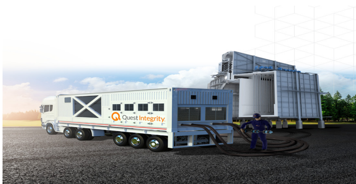
Figure 4. Set up for coil cleaning and inspection (typical process heater).
